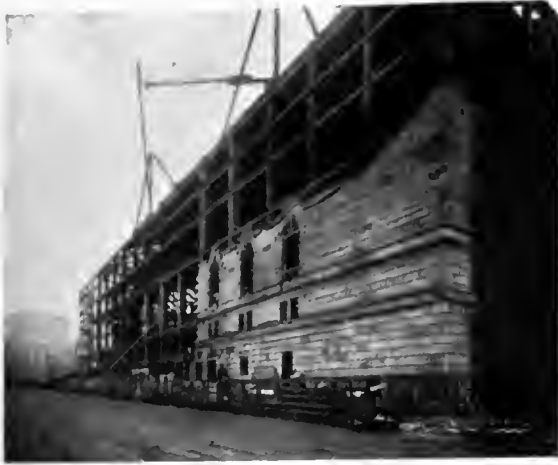
RECENT PROGRESS VIEW SHOWING STONE-WORK OF MAIN FAÇADE WELL UNDER WAY
